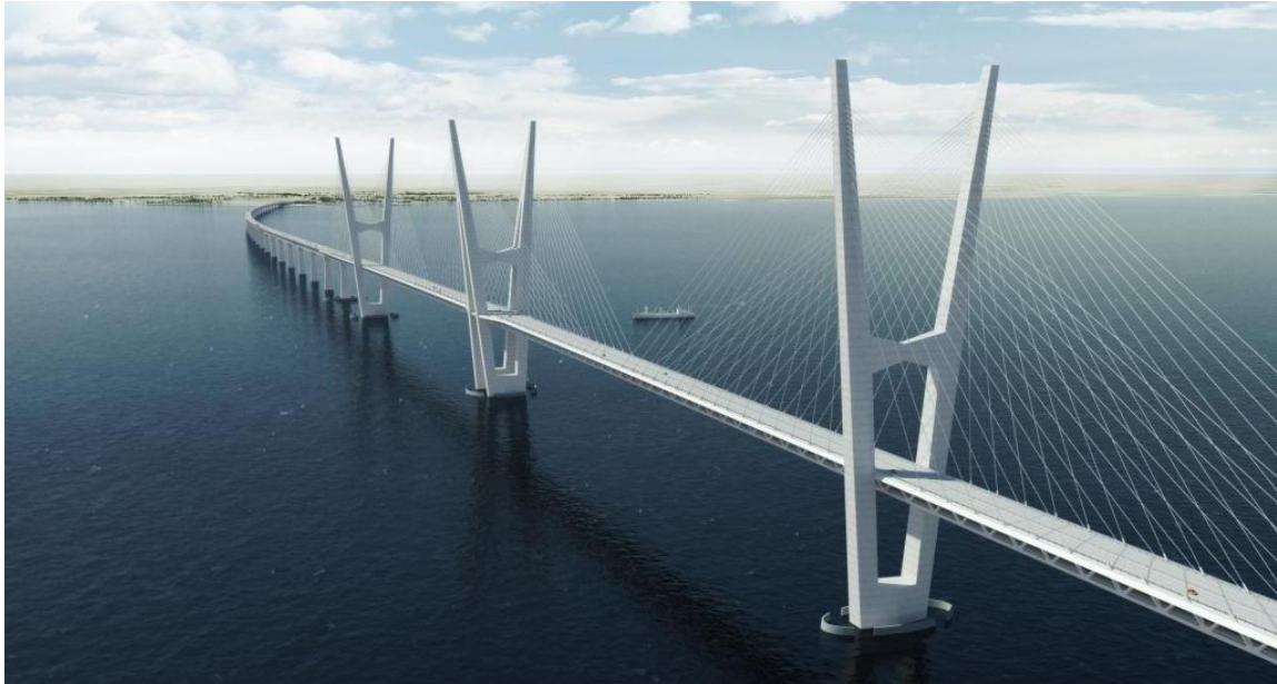
Perspective of a high bridge across the Fehmarnbelt with two free spans of 724 m each.
