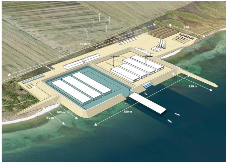
Theoretical illustration of a traditional production facility for tunnel elements
